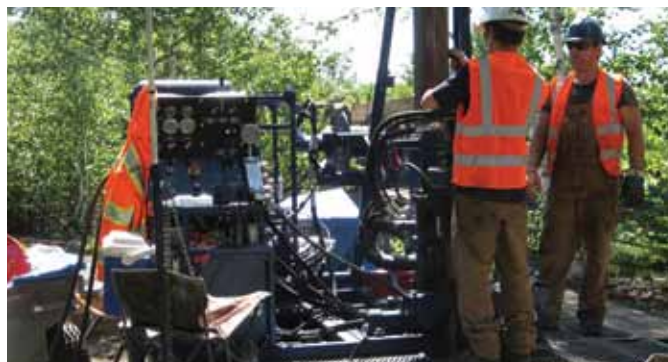
→ Above: Diamond Drilling, Long Lake
