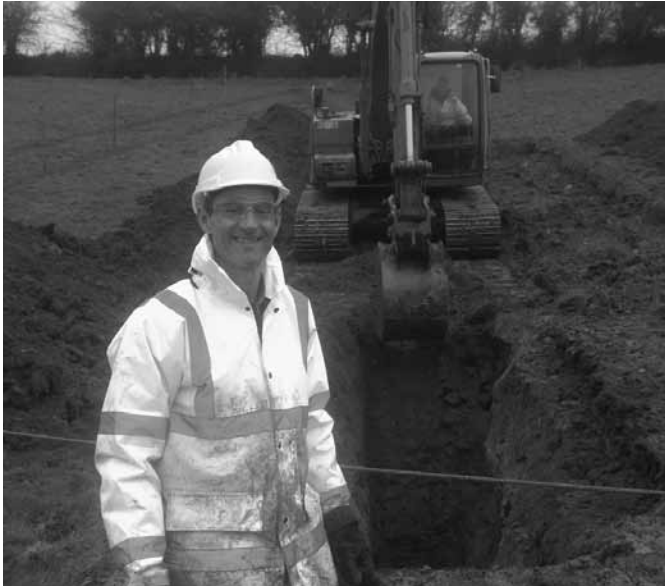
→ Above: Trenching at Derryginagh 2010.
