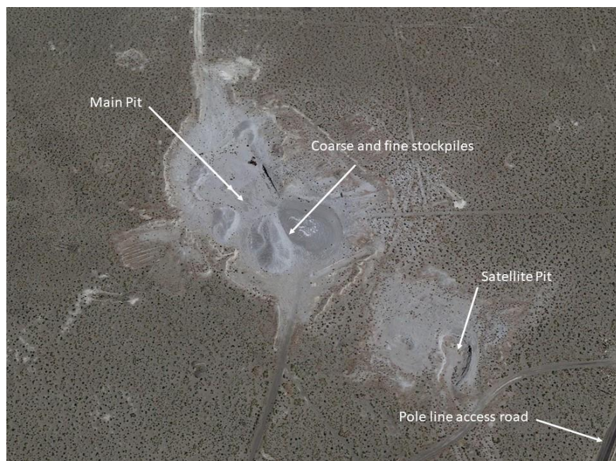
Figure 12: Open pits at the Hazen Project
